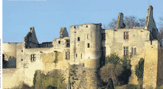
BEFORE: Chinon before restoration
